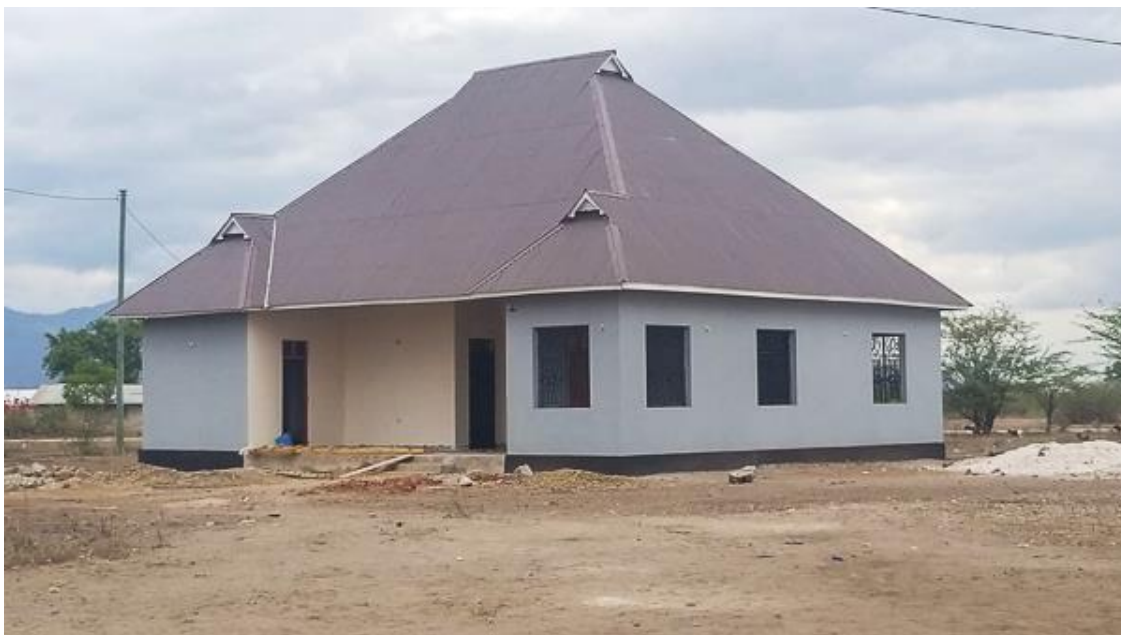
"Toloha Training Center", Bauzustand Juli 2022
